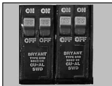
(E) Verify circuit breaker not tripped; if it is tripped, reset it once only.
