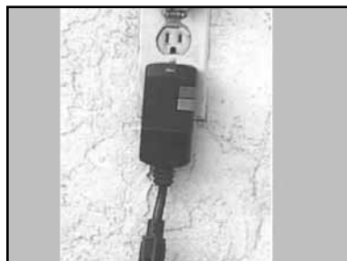
(E) Unplug the GFCI from the Power source.
