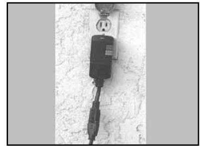
(C) Check to see if the Ground Fault Circuit Interrupter (GFCI) tripped.
