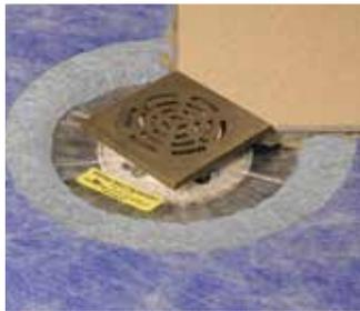
Installed in a thin-bed method shower with NobleSeal® TS waterproofing membrane, NobleFlex Drain Flashing®, and Positive Weep Protector™.
