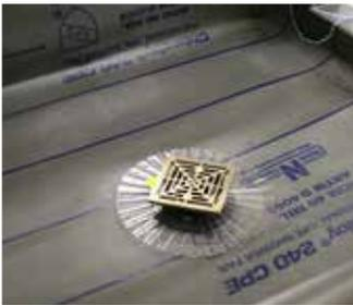
Installed in a full mortar bed method shower with Chloraloy® shower pan liner.
