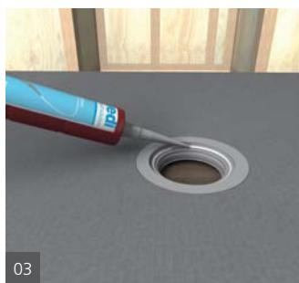
**EN** Set up a continuous 1/4" bead of wedi Joint Sealant along the top side of the wedi Fundos' valve groove profile.
