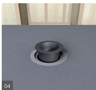
**EN** Drop the drain body firmly into the sealant.
