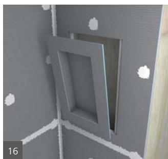
**EN** 2 Fasteners each side of the niche are set to create a flush transition to the wall panels. Another 1/2" bead of wedi Joint Sealant is spread over fasteners and seams.
