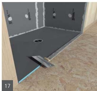
**EN** Apply thinset mortar over wood subfloor and reaching 4" into the wedi Fundo Ligno shower base. Fill the wedi Fundo Ligno channel with thinset or a strip of sealed on wedi Building Panel and apply thinset mortar to the lower corner of the wedi wall panels left and right of any entrance using 1/4" x 1/4" notch trowel.
