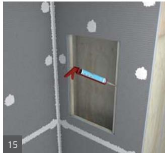
**EN** wedi Niches are installed in a cut out in the wedi wall and attached with it's flange right into the center of 16 o.c. studs. wedi Joint Sealant is set along the connection of wall to niche.
