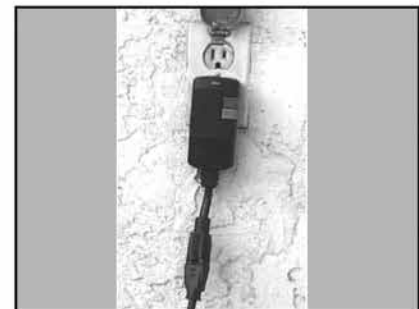
(C) Check to see if the Ground Fault Circuit Interrupter (GFCI) is tripped.
