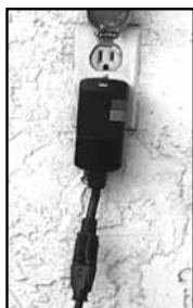
(A) Unplug GFCI from BX-3 and power source.
