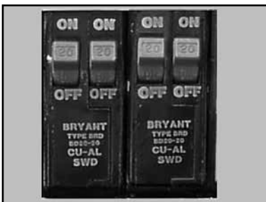
(D) Verify the circuit breaker is at least 20 amps – if not, move to 20 amp circuit.
