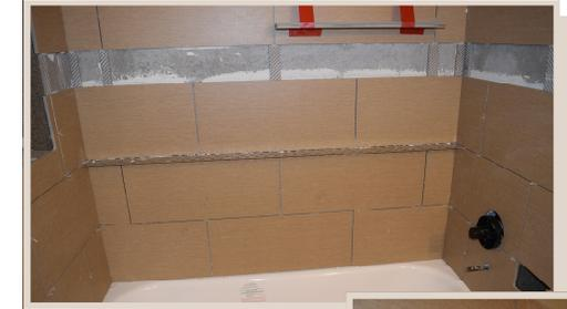
**4.** Place the *Ledgeline™* directly on top edge of selected tile course. Apply surface bull-nose tile (SBN) or other finish material to top and bottom of *Ledgeline™* by using thin-set or mastic to "sandwich" shelf unit. Allow front edge of applied tiles to extend 1/8" minimum to allow for grout coverage of shelf.
