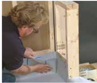
Fold corners and fasten upturns to studs
