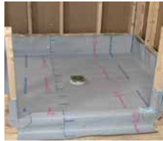
Completed in minutes
