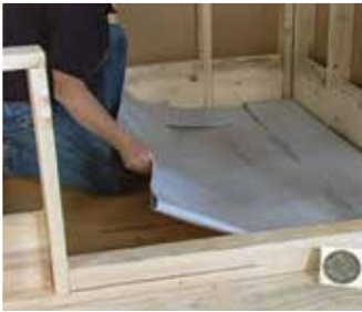
Install Chloraloy allowing for upturns
