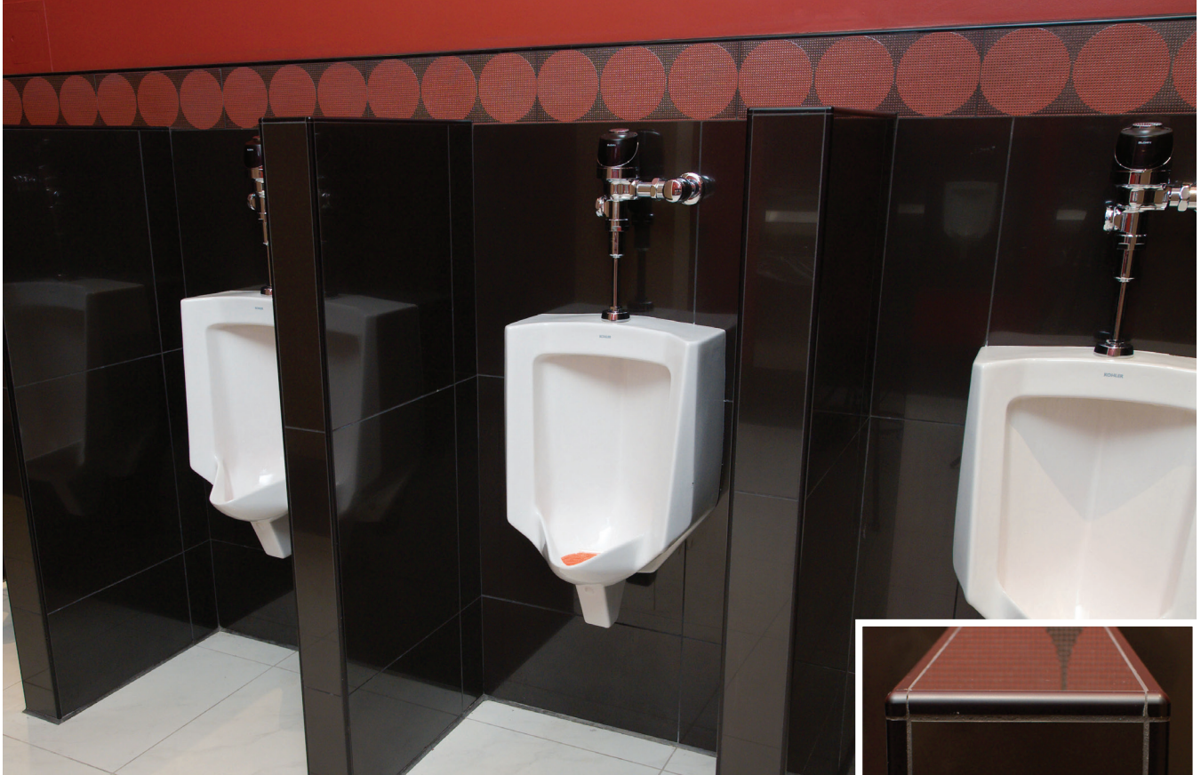
RONDEC bullnose profile and corner piece accessories in brushed black applied to the tile edges on the walls and partitions.
