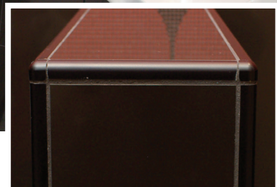
RONDEC bullnose profile and corner piece accessories in brushed black applied to the tile edges on the walls and partitions.
