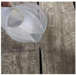
5. After brushing, flush the Drain Channel with several gallons of warm water.
