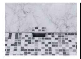
Re-Install the Access Cover Tray by angling the cover down to the Drain Channel until the ball detents catch the Access Cover Frame. Push the cover down until flush.
