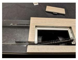
4. Use the round Brush to clean the Drain Channel. The metal portion of the brush head can be formed as needed to access the Drain Channel more effectively.
