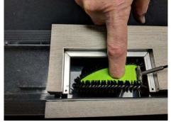
3. Holding the D-shaped Brush with your finger, lower the Brush into the Access Opening with the straight side parallel to the Drain Channel. Push the Brush forward into the Main Channel and pull back and forth several times to clean. If possible, avoid rubbing the Brush shaft on the lower perimeter of the Access Cover Frame.
