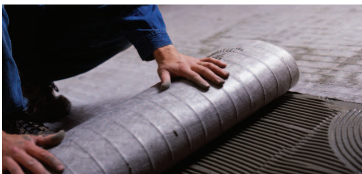
FIGURE 2.13: Place mat onto fresh thinset
