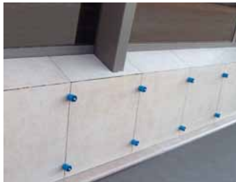
T-shaped leveler installation.
