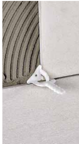
T-shaped leveler installation.
