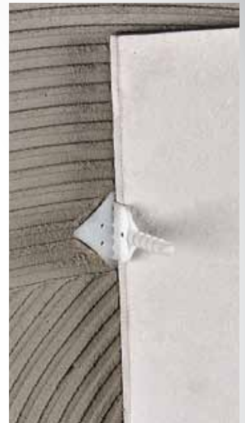
Linear leveler installation.
