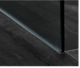
JOLLY offers a discreet and minimalist reveal to elegantly frame the elongated niche. DILEX-EKE eliminates the need for grout and separates the individual tile fields at the floor/wall transition. DECO-SG acts as a support channel for the glass wall.
