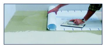
**3.** Using the flat side of the trowel, press the mat into the thinset ensuring that the mat is free of air pockets and crimps in the fabric. Start at one end and continue working in one direction to avoid air pockets.
