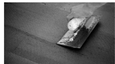
**Normal installation conditions - apply bond coat. Trowel an area as wide as the sheet and as deep as can be comfortably reached (comb ridges parallel).**
