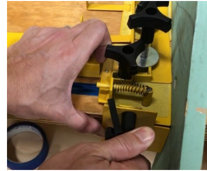
Figure 4: Locking in plates flush with wall
