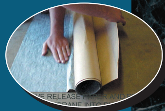
Remove & Press in Place
