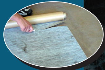
Cut to Correct Length
