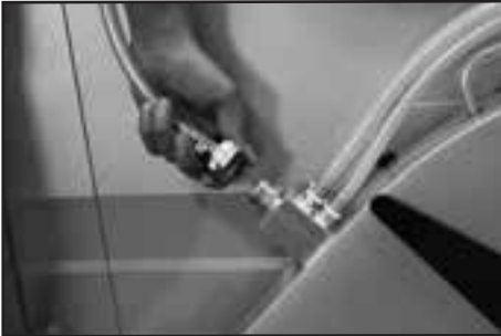
Fig. 5 Unscrew Hose Fitting
