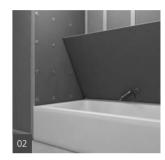
Attach a notched panel to the framework with a 1/2" bead of wedi Joint Sealant between the notch and flange. Attach the panel to the framework using wedi Washers and Screws at a rate of 1 every 12 inches along the studs. Leave a gap of 1/8" between tub edge and wedi panel bottom end to allow for movement of the tub. Alternatively apply a bead of wedi Joint Sealant in between both materials.
