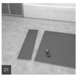
Measure and cut wedi Building Panel to fit the 16 inch o.c. framework (wood or metal). Notch out all panels if installed around the perimeter of a flange tub to integrate the flange and achieve a plumb wall with square and tight corners.
