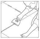
Remove all debris from panel surfaces; vacuum carefully to eliminate excess dust and dirt.
