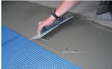
2. The type of thinset mortar used to apply BLANKE PERMAT must be appropriate for the substrate in accordance to the manufacturer's recommendations. Apply loosely-mixed thinset mortar to the substrate using a notched 1/4" x 1/4" trowel. The consistency should be slightly more liquid than normal to allow for absorption into the fleece underside of the mat.
