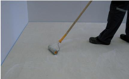
1. Substrates must be clean, load bearing, and free from non-adhesive substances. Please refer to the most recent TCNA Handbook for Ceramic Tile installation for further details regarding current standards of application.
