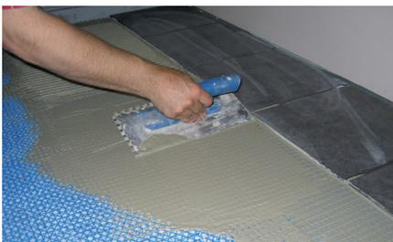
7. Fill the cavities of the fiberglass mesh evenly with thinset mortar. Then apply sufficient thinset mortar to the area, wet-on-wet, then comb using a notched trowel appropriate for the tile or stone installation.
