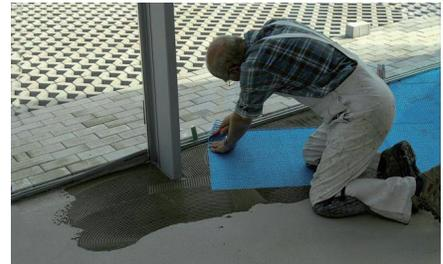
6. Cut BLANKE PERMAT to the correct size with scissors or knife as needed to fit flooring surface.
