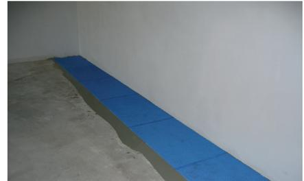
3. Do not install BLANKE PERMAT flush against a vertical surface (ie wall or support column) - instead leave a 1/4" gap between the mat and any restraining surface ie; wall, cabinet toe kick, stair riser. Use a knife to cut off any excess mat. Lay BLANKE PERMAT starting at the corner from right to left so the panels overlap fit together cleanly.
