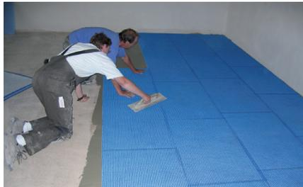
5. Embed the underside fleece (white side down) into the fresh thinset mortar so that its entire surface is bonded. Press the mat into the mortar by using a float or a roller. You must offset the joints of BLANKE PERMAT by at least 4".
