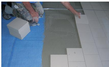
8. Allow tile to cure per manufacturer recommendations before grouting. Typical wait time is 24 hours.
