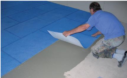
4. BLANKE PERMAT sheets have a mesh overhang of approximately 1" on two adjoining sides. These overhangs are needed to join the mats at their seams. It is not necessary to further reinforce the joints of the mats. Butt the mats tightly against each other and avoid any gaps between sheets.
