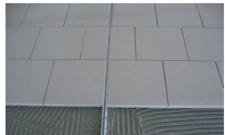
9. Expansion and movement joints must be installed where specified. We suggest using Blanke Expansion Joints for this purpose: BLANKE FLOOREX, BLANKE Surface Expansion Joint, or BLANKE Heavy Duty Expansion Joint.
