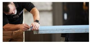
A wedi shower base can be cut to size using a circular saw with standard carbide blade. You can remake the 1/2 inch x 1/2 inch perimeter channel by cutting through the cement surface using the circular saw set to cut 1/2 inch deep. You can use a circular saw or a sharp utility knife to cut the new channel 1/2 inch wide through the blue exposed foam side. Clean the new channel and the base and remove all saw dust and loose particles.
