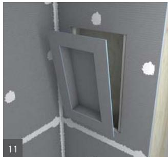
**EN** 2 Fasteners each side of the niche are set to create a flush transition to the wall panels. Another 1/2" (13 mm) bead of wedi Joint Sealant is spread over fasteners and seams.
