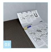
Insert wedi<sup>®</sup> Subliner Dry with the printed side facing upward and press on with a rubber roller or wooden float. Remove air pockets and other foreign particles from below the sheets.
