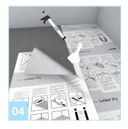
The sheets must overlap 2" (50.8 mm) at joints/transitions. Leave these overlapping areas free of any thinset and use tape to keep them folded upward and/or clean. Once the thinset has cured, apply wedi® Sealant 620 as a full bed onto the lower mat's seam connection area and press the top overlap flap into the wedi® Sealant 620.
