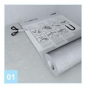
Lay out wedi<sup>®</sup> Subliner Dry and cut to size using a knife or scissors.
