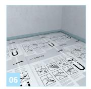
In complete wet rooms, wedi recommends to flash Subliner Dry up the wall by 2" (50.8 mm) where it is still invisible behind the baseboard tile or wood applications.
