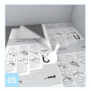
Spread all the wedi<sup>®</sup> Sealant 620 flat using a putty knife. Cross joints should be avoided.
