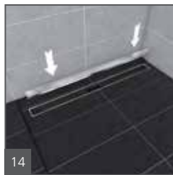
14 Insert the wedi drain cover.
