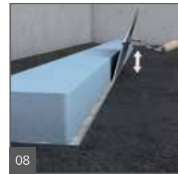
08 Apply thinset mortar to support the profile at desired height.
